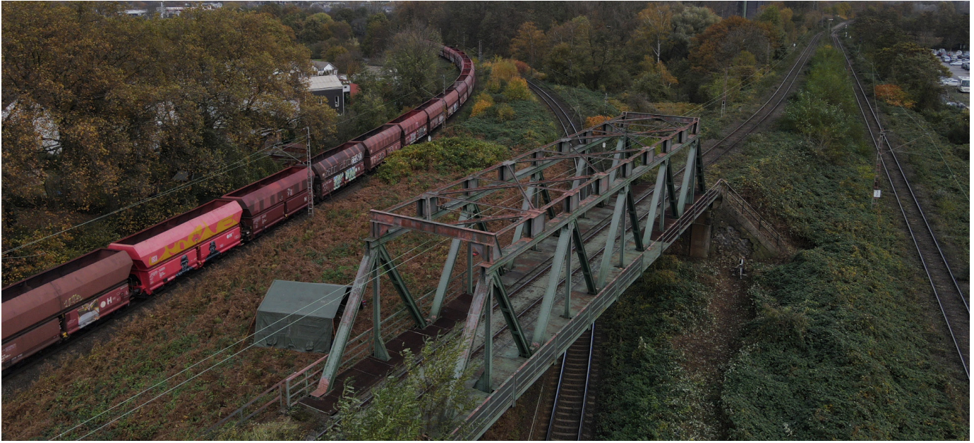
Precision Metrology in Action - Hilmar Schroeder and Christian Sommer collaborate to scan the 60-year-old steel bridge with high-accuracy equipment.
